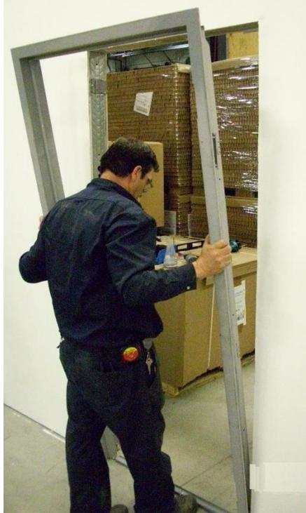
**Figure 6 : *Placing the frame into the opening***
