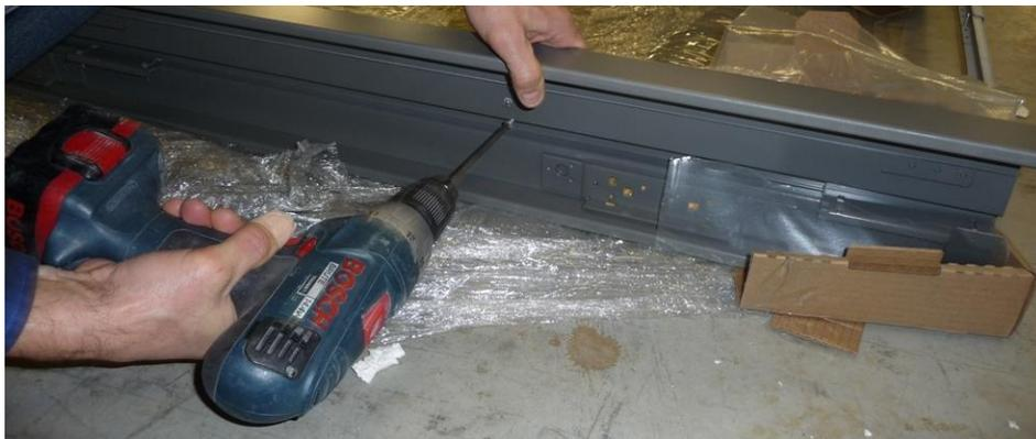
**Figure 5 : Removing the shipping screws**
