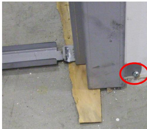
**Figure 8 : Screwing the strap anchor**
